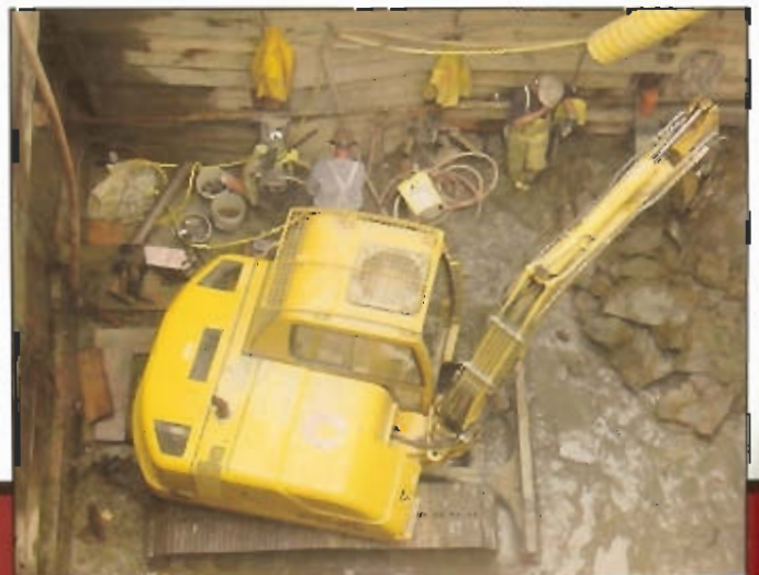
Excavation of the 100 foot deep drop shaft
